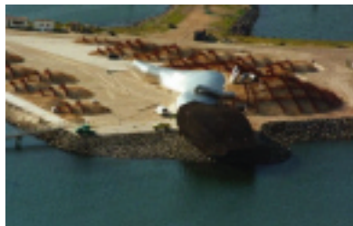
The Water Pavilion - the Salt Water side by Oosterhuis in the front and the Fresh Water side by Spuybroek in the back.
